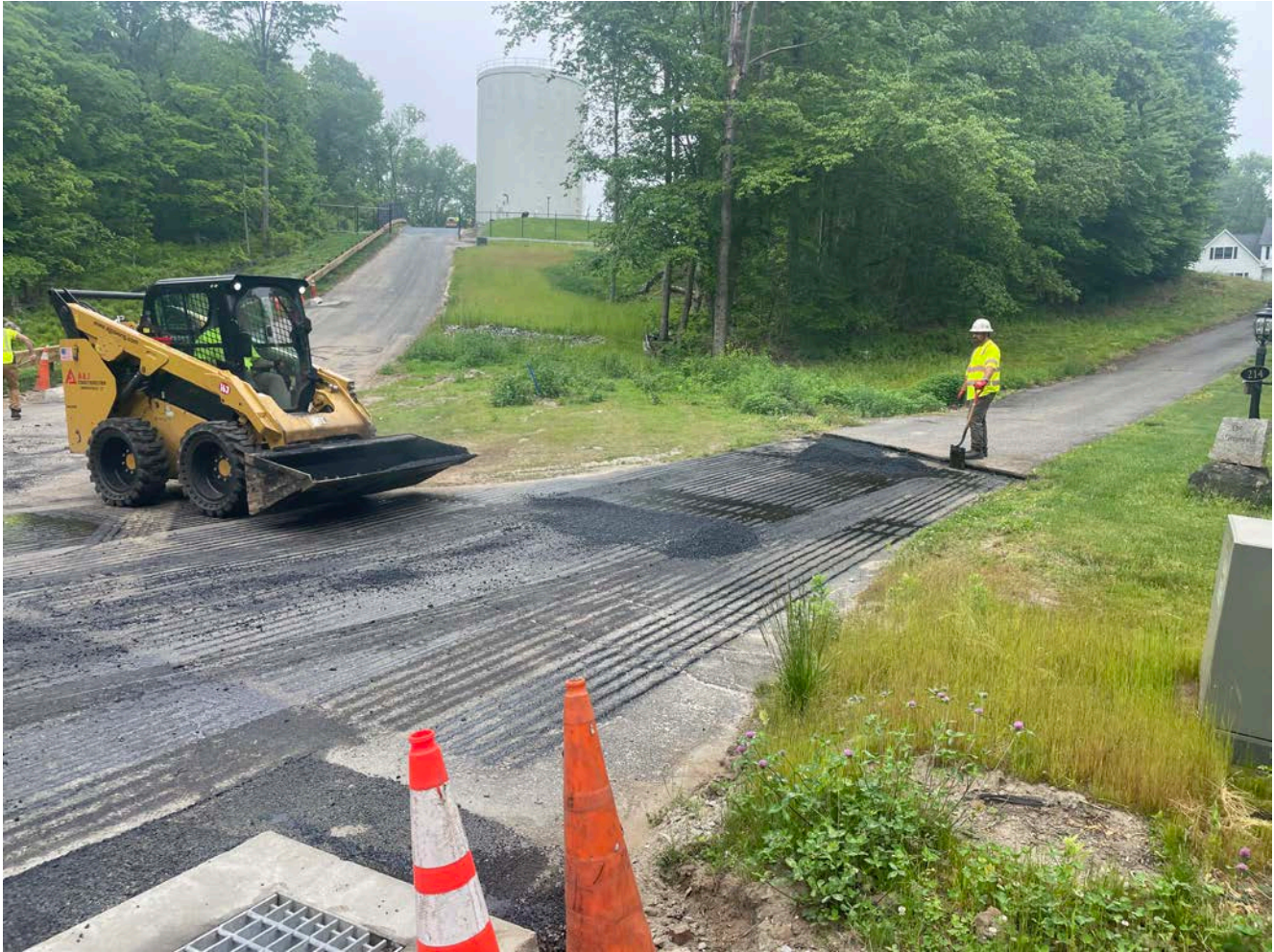
Picture 5: A&J Construction about to place asphalt on the driveway apron for the 224 Talcott Ridge Drive property after having placed tack coat. View to the east.
