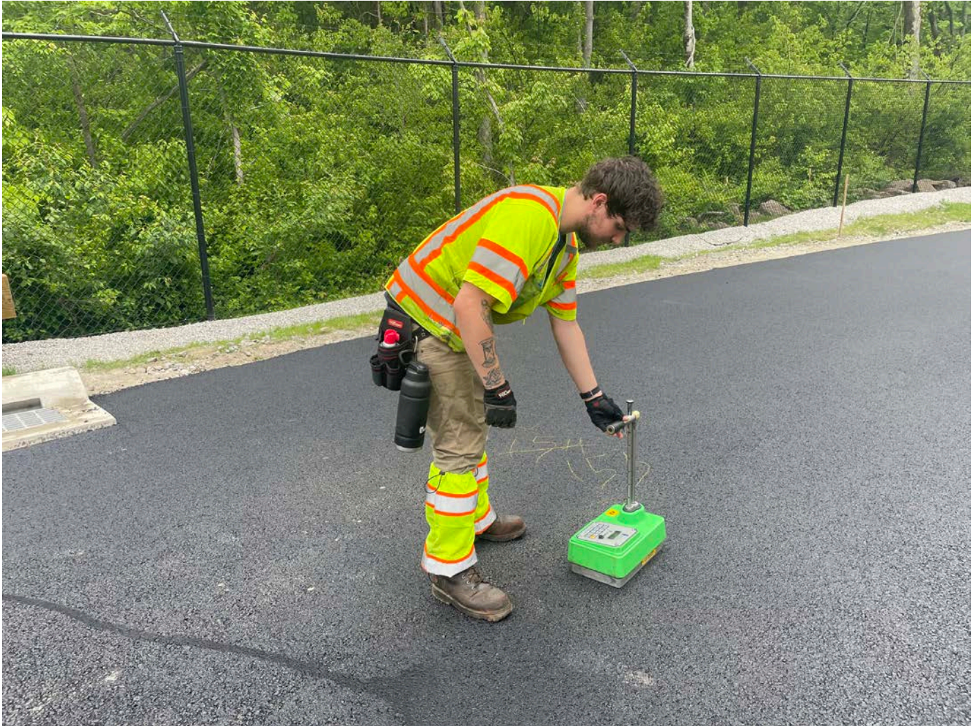
Picture 9: Advanced Testing checking temperature and compaction on the asphalt that A&J Construction placed at Station ~10+50 on the Shared Access Driveway. View to the northeast.
