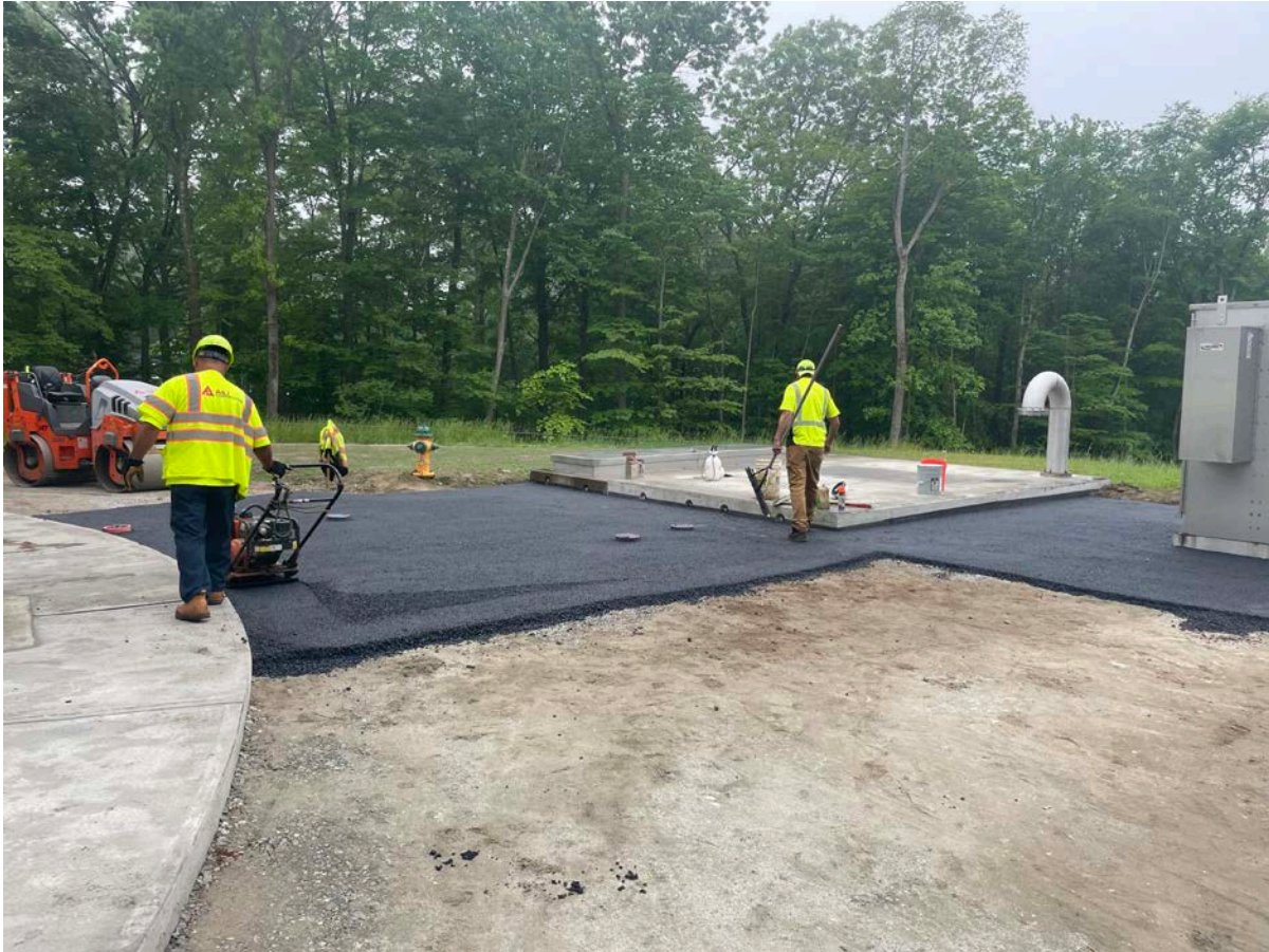
Picture 1: A&J Construction placing the first lift of asphalt around the electrical enclosure located on the west side of the water tank located on the east side of the Shared Access Driveway. View to the southwest.
