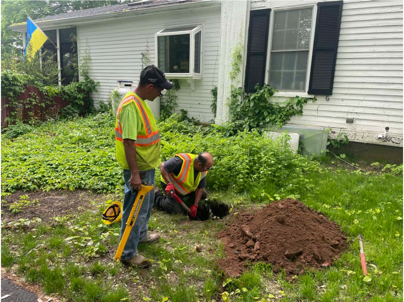
Picture 4: Ludlow locating the well on the north side of the 313 Main Street residence. View to the southeast.
