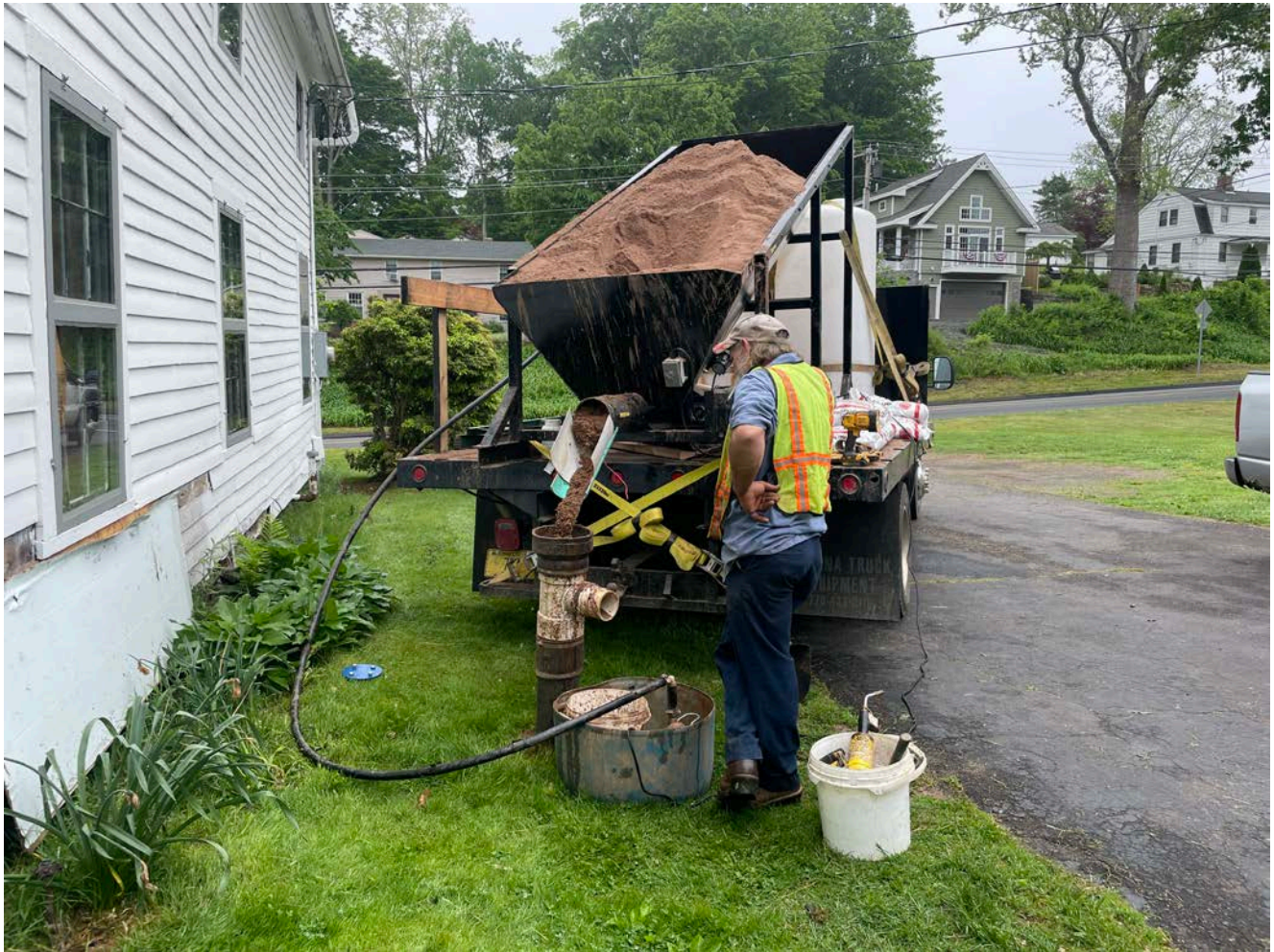
Picture 2: Grela placing sand into the well located on the north side of the 167 Main Street, Durham, residence as part of well decommissioning activities. View to the west.
