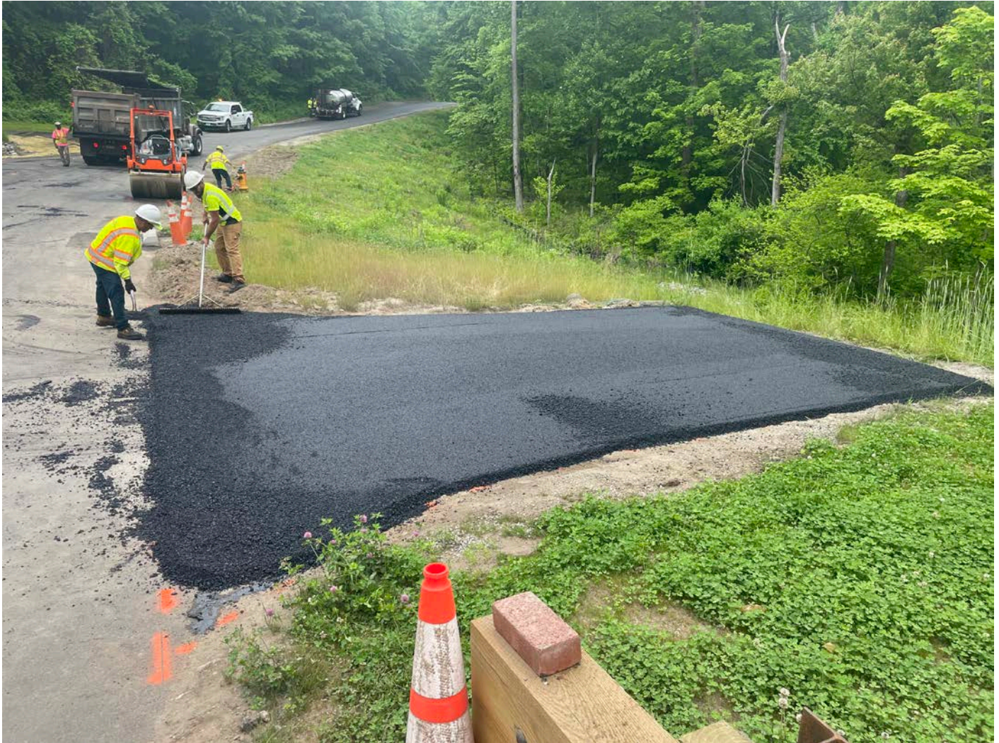
Picture 6: The turn out located at Station ~14+00 on the Shared Access Driveway where A&J Construction just placed a lift of asphalt. View to the west.
