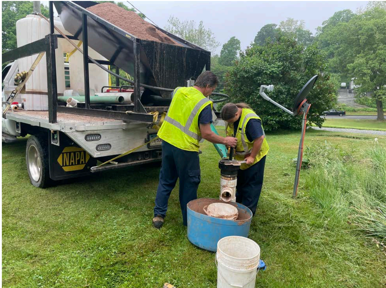
Picture 3: Grela placing sand into the well located on the south side of the 177R Main Street, Durham, residence as part of well decommissioning activities. View to the west.
