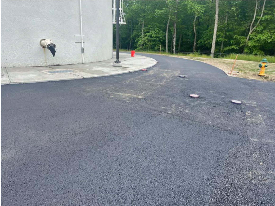
Picture 7: The south side of the water tank where A&J Construction just placed the first of two lifts of asphalt. View to the south.
