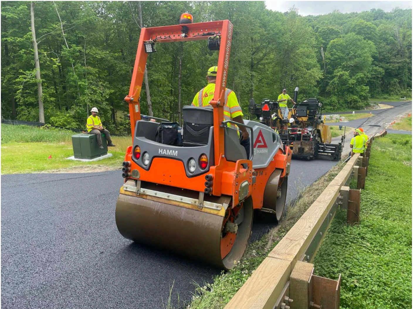
Picture 16: A&J Construction placing and rolling asphalt on the Shared Access Driveway. View to the west.
