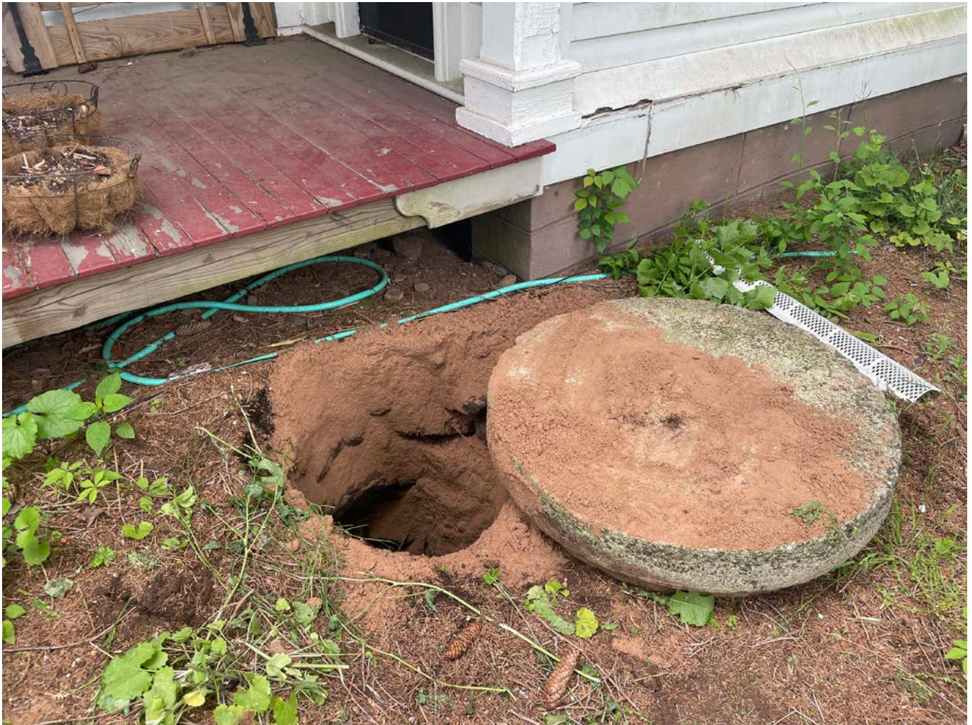
Picture 14: The dug well located on the south side of the 313 Main Street residence that Ludlow daylighted in order to allow Grela to decommission the well. View to the north.
