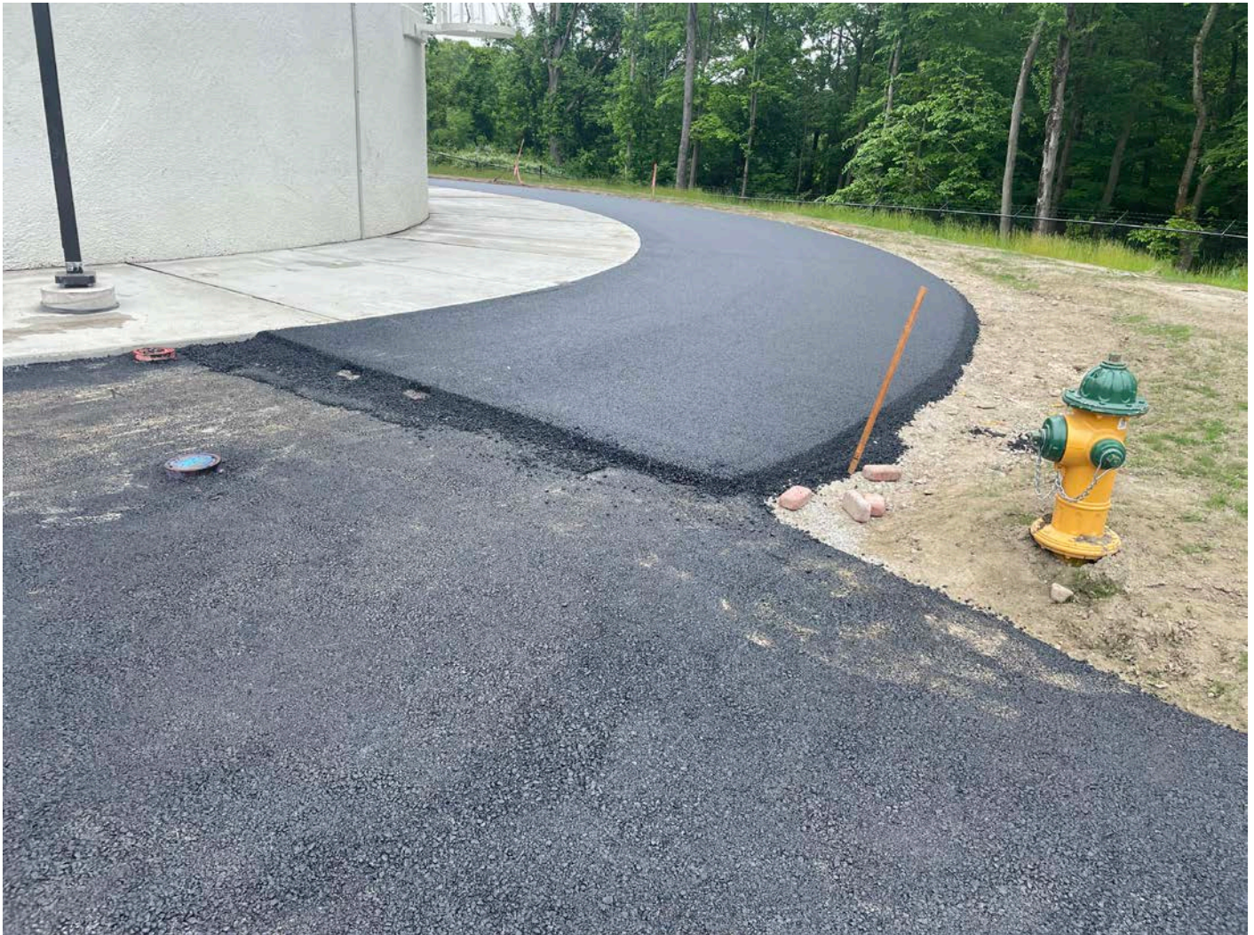
Picture 12: The south side of the water tank where A&J Construction is in the process of placing the second of two lifts of asphalt. View to the southeast.
