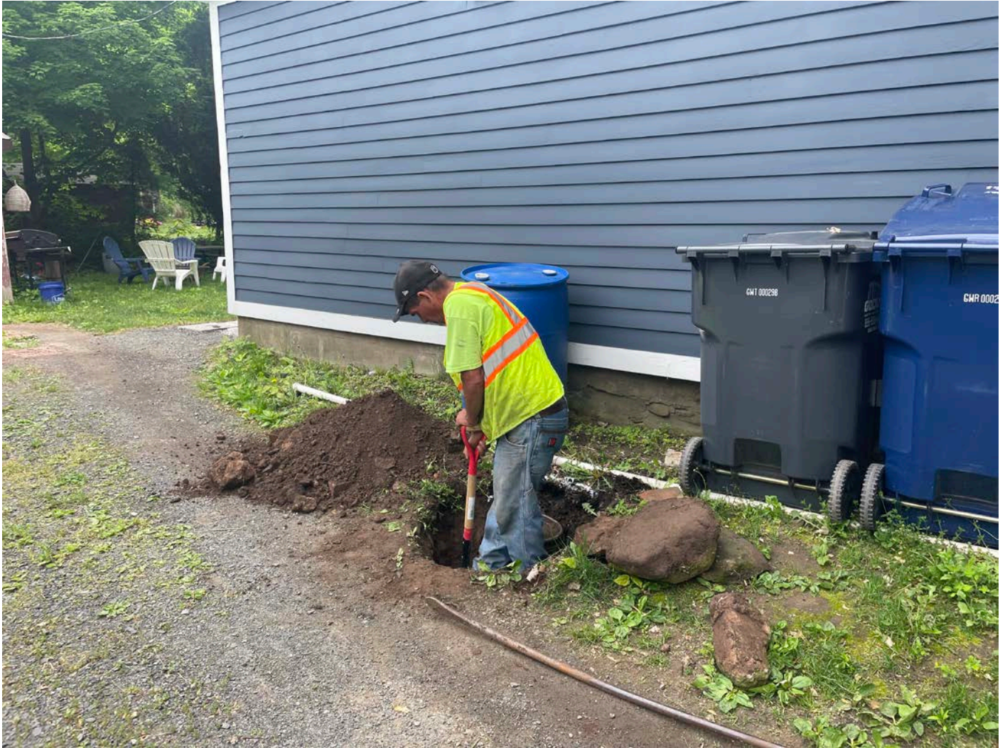
Picture 13: Ludlow excavating around the well casing on the north side of the 271 Main Street residence. View to the southeast.
