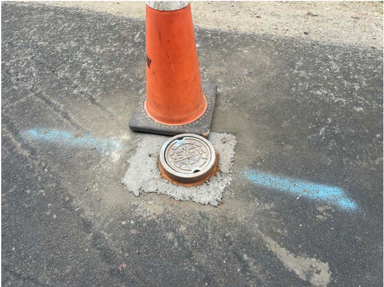
Picture 10: Station 17+91 where Ludlow placed concrete around a road box they raised. View to the northwest.
