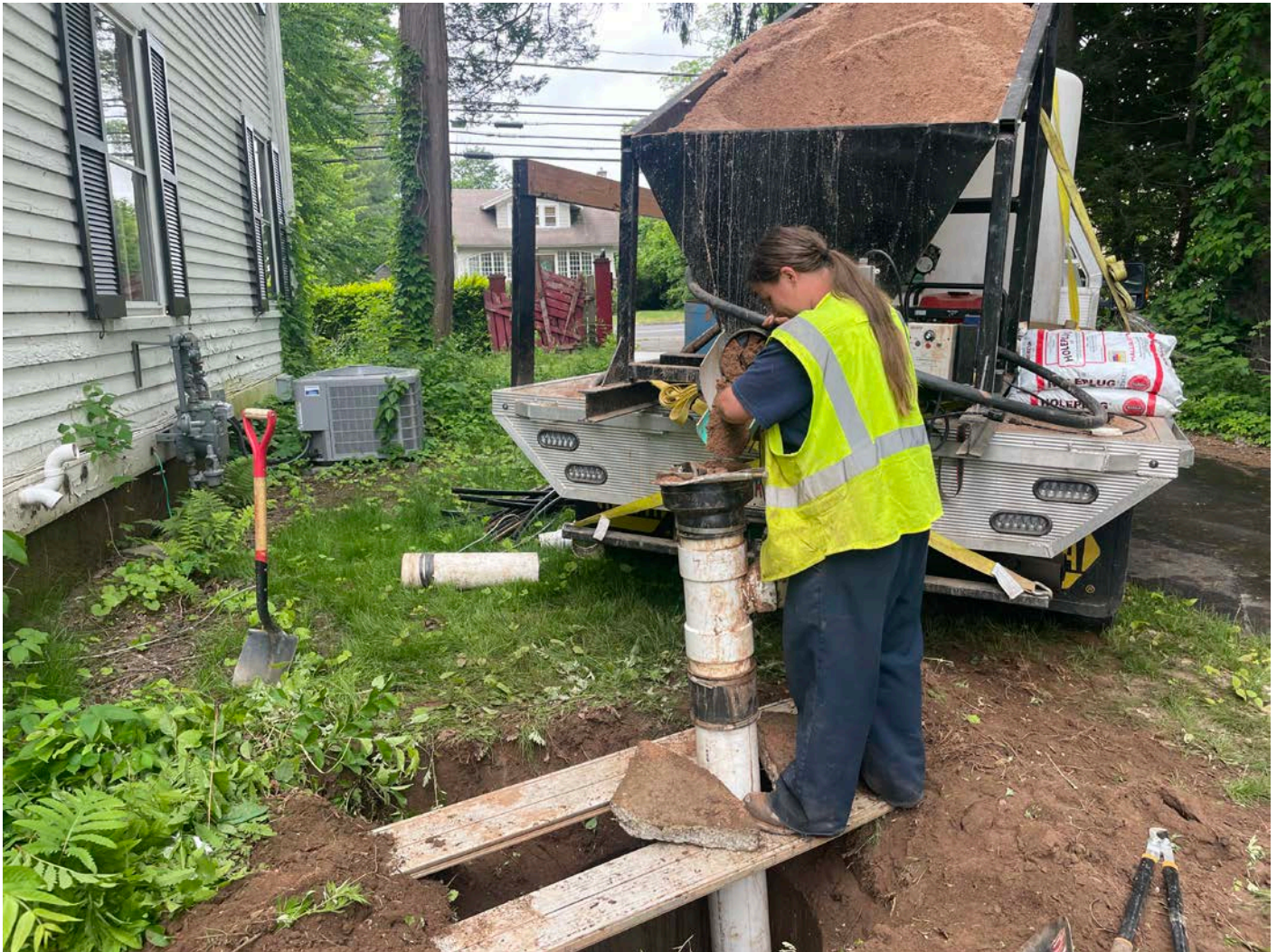
Picture 15: Grela placing sand into the well located on the north side of the 313 Main Street residence as part of decommissioning activities. View to the west.
