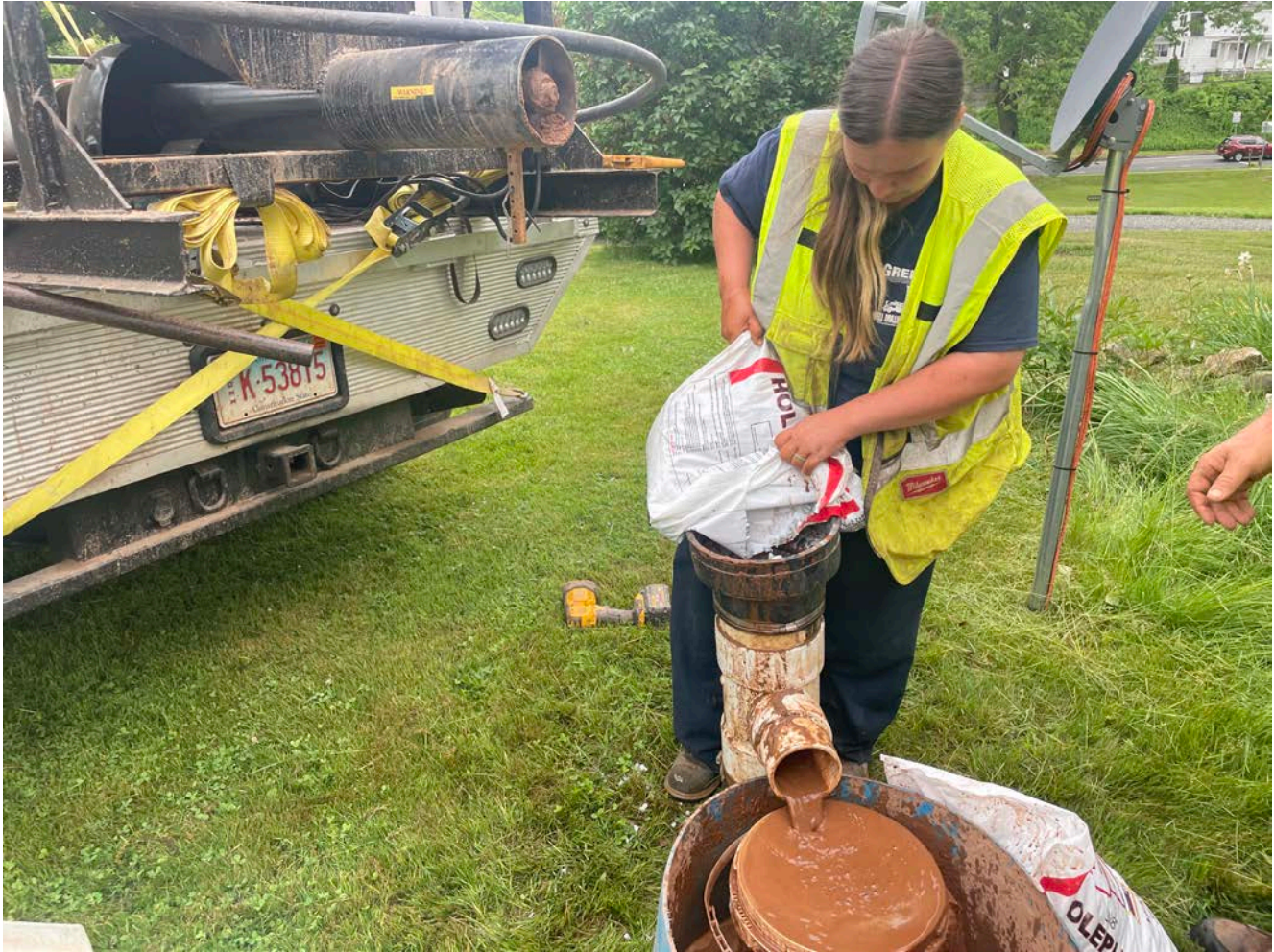
Picture 11: Grela placing sand into the well located on the 177R Main Street, Durham, property as part of well decommissioning activities. View to the west.
