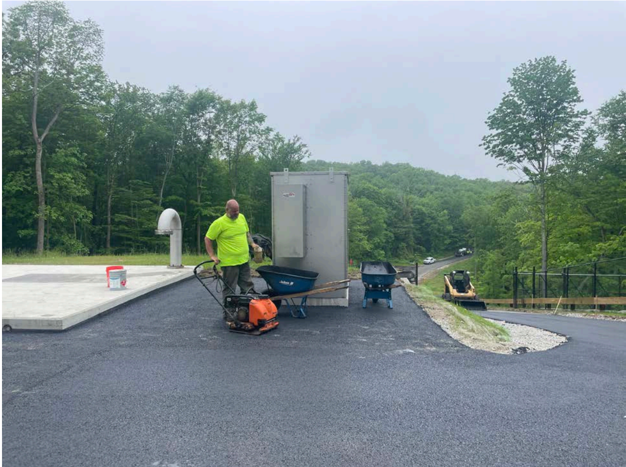
Picture 8: The electrical enclosure located on the south side of the water tank where A&J Construction just placed the first of two lifts of asphalt. View to the west.
